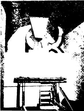
circulation and venting arrangement of a 400 cubic meter railroad disinfestation chamber
