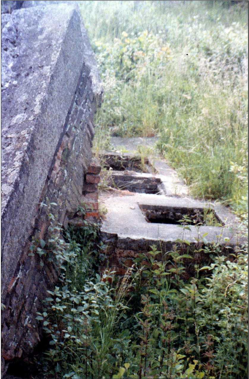
Photo 9: Inspection shafts in the ruins of Crematorium III at Birkenau. © C. Mattogno.
