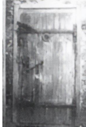
Delousing gas chamber doors in Auschwitz: The same picture over and over again: Wooden doors of normal size, provisionally made gas-tight. (J.-C. Pressac, Auschwitz:... , op. cit., pp. 48, 50)
