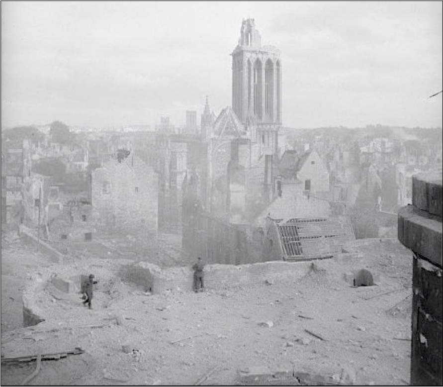
A general view of Caen showing the extensive damage caused by Allied bombing, 9 July 1944. By No 5 Army Film and Photographic Unit, Stewart (Maj) [Public domain], via Wikimedia Commons
