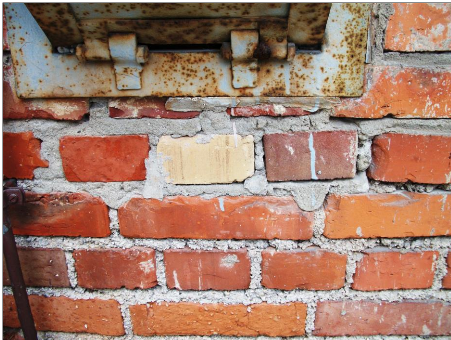
Photo 18: Mortar variation in right chute.
