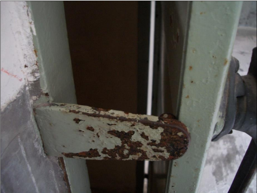
Photo 10: Exit door obstruction.
