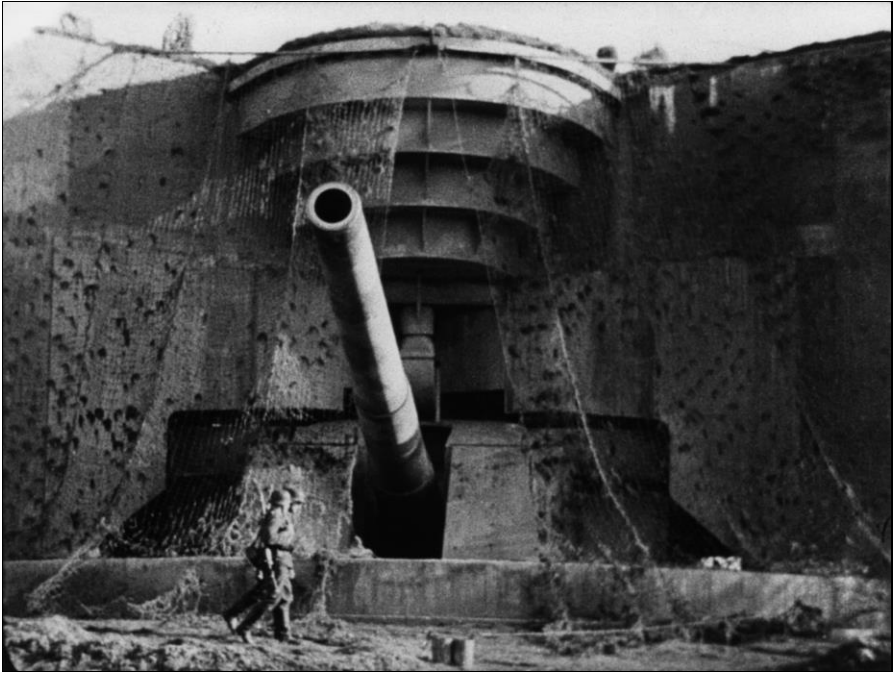
A coastal battery with camouflage netting. During the Normandy invasion, four battleships bombarded a similar gun position at Houlgate. The battery sustained over 1,000 hits, some from 15-inch diameter projectiles and from aerial bombs, without serious damage.
