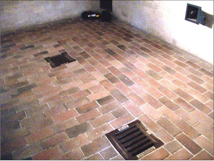
Photo 3: Gas chamber floor.
