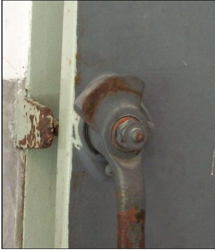
Photo 9: Exit door obstruction.
