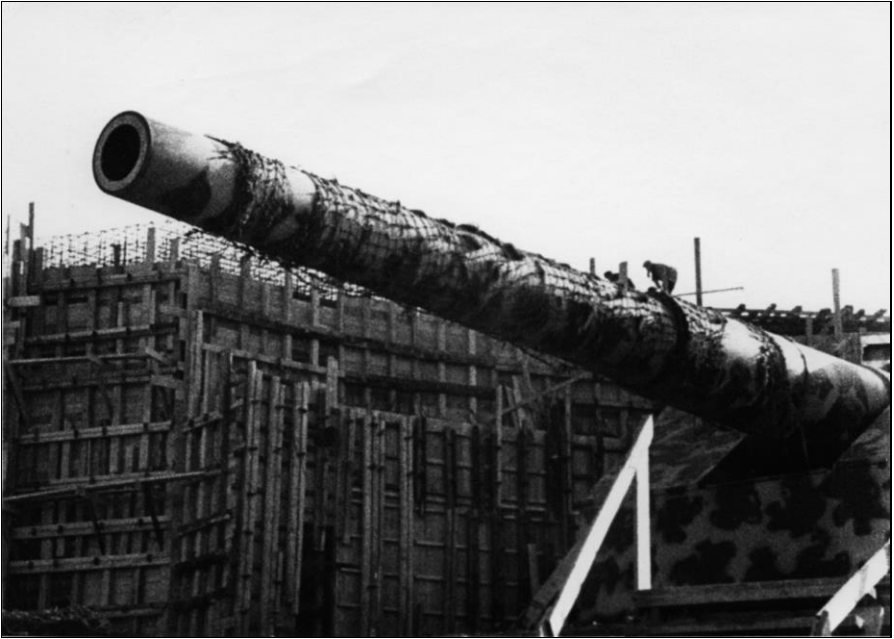
Battery Lindemann along the Atlantic Wall. The Germans constructed massive concrete shelters to protect coastal artillery from damage by Allied aerial and naval bombardment.
