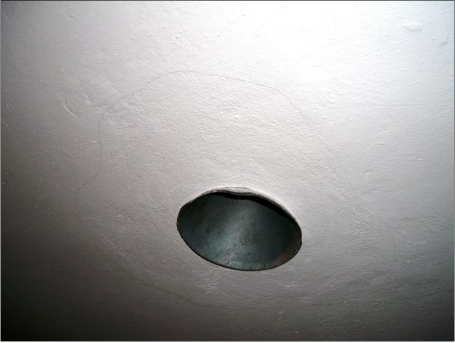
Photo 7: Rework to ceiling around shower head.
